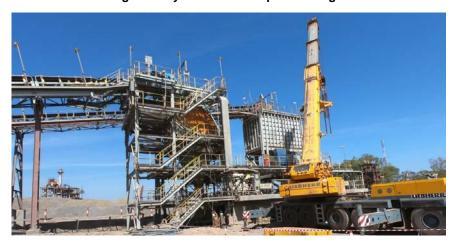
Figure 5: Syama Sulphide crushing circuit - new HP5 crusher installation
