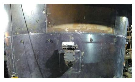
Figure 2: Syama Roaster steel replating
