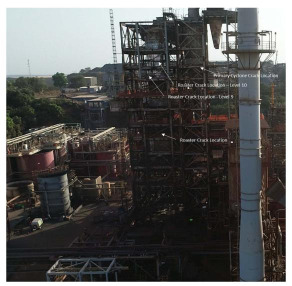
Figure 1: Syama Roaster showing repair locations
