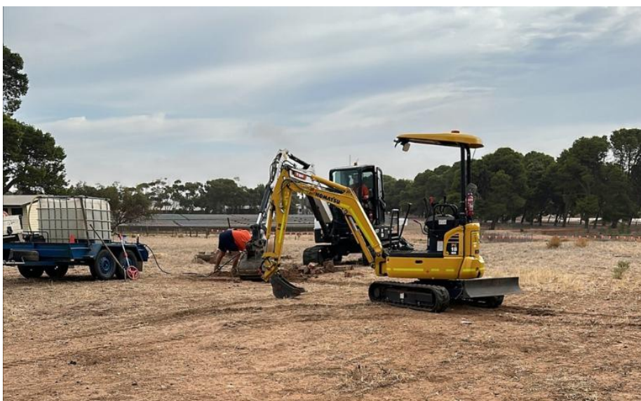
Figure 1: Site preparation activities, Roseworthy, South Australia
