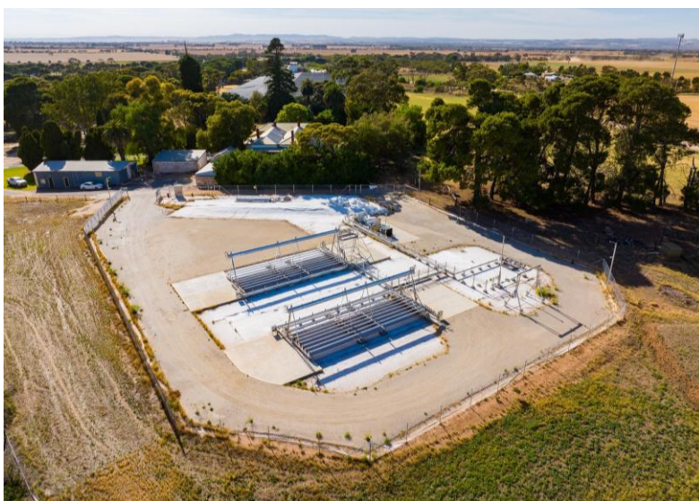
Figure 2. Sparc Hydrogen's SHARP Pilot Facility at Roseworthy, South Australia
