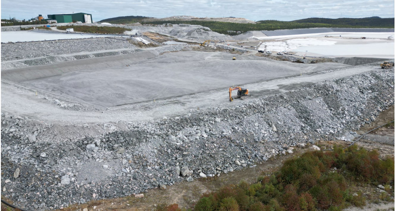
Figure 4: Earthworks around Tailings Storage Facility 1
