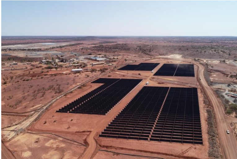
Figure 3: Westgold Resources Limited recently commissioned hybrid power station in Cue
