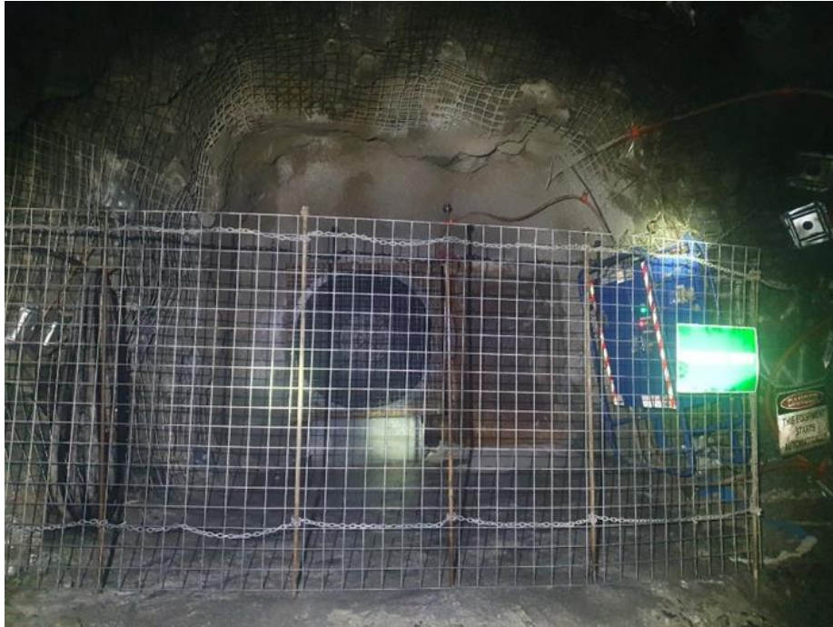
Figure 4: New ventilation fan station set in shotcrete ground support.
