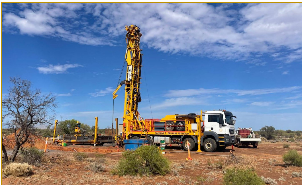
Figure 2. Core drilling at the Byro REE Project
